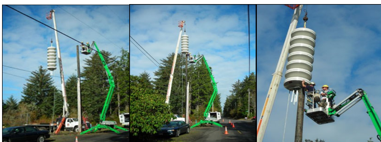
AHAB Siren being installed on U Street in Ocean Park.
