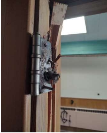
The aftermath of a ballistic breach on a commercial door hinge
